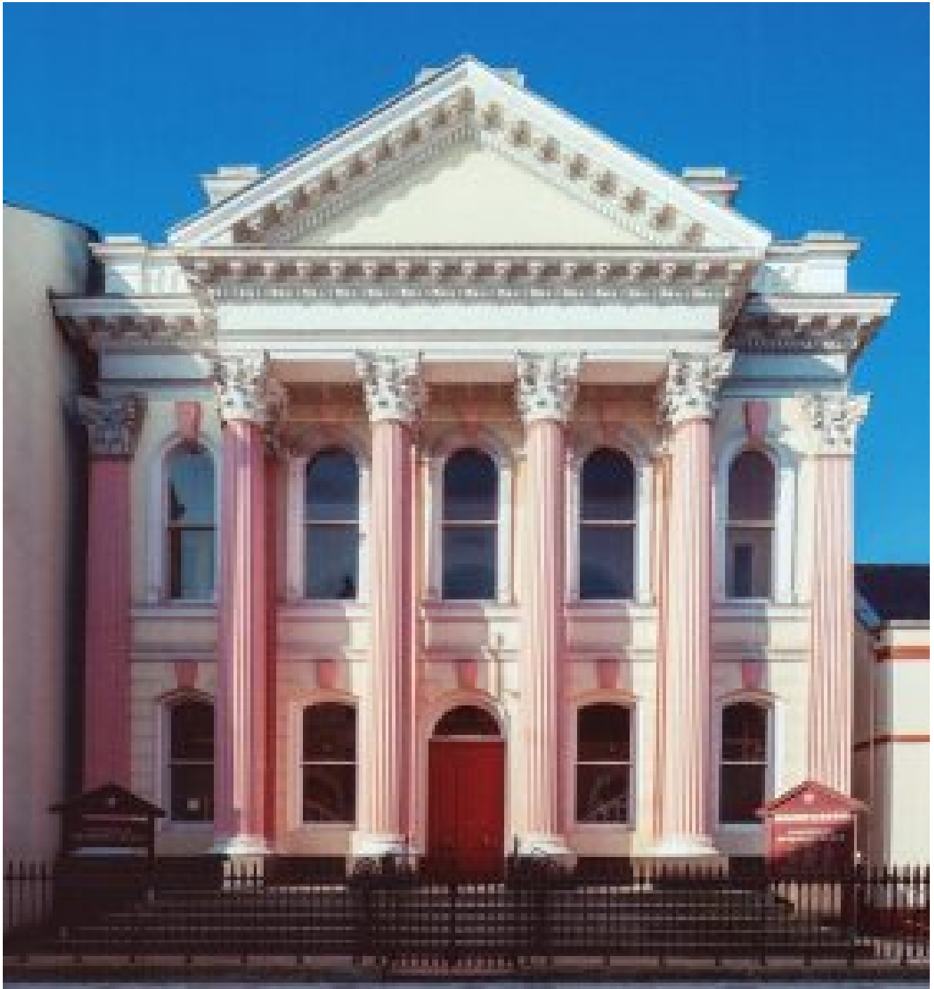
Figure 12: Confident Roman Corinthian temple-front of the Methodist Church, Darling Street, Enniskillen, County Fermanagh (1863-5).
