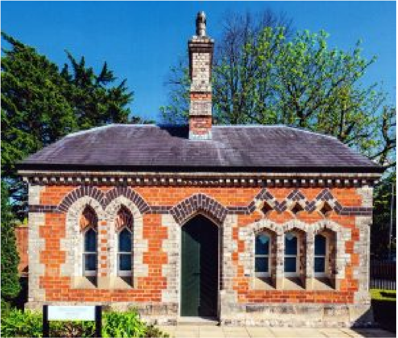
Figure 13: Former gatelodge for Belmont Presbyterian Church, Belfast (1860-1), showing the beautifully considered complex polychrome treatment.
