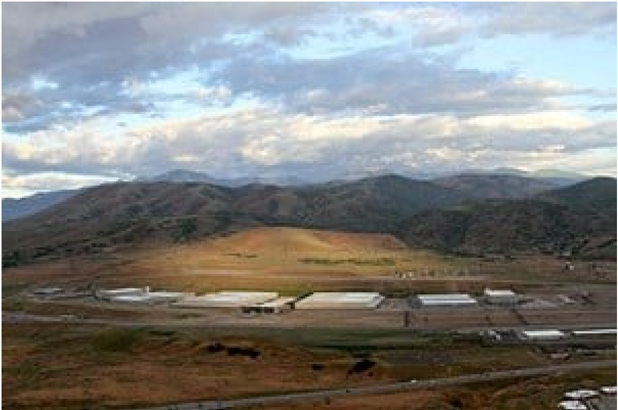
Bluffdale Data Center, Utah
